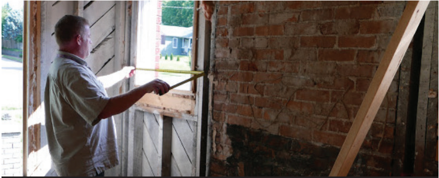
Inspector Fred Zahn, in Nashville, Tennessee, checks the reframing of a window during a major rehab.
